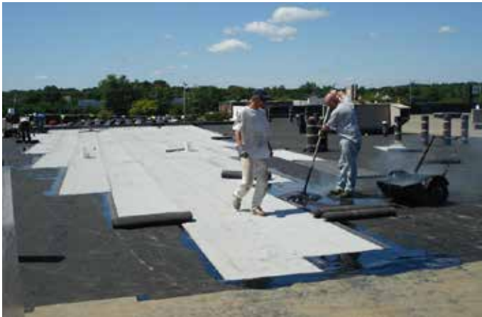
Built-up roof system – A commonly used flat roof system
