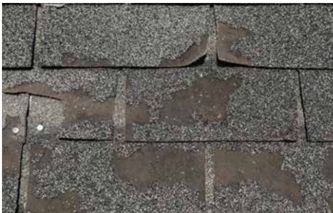
Example of granule loss on asphalt shingle
