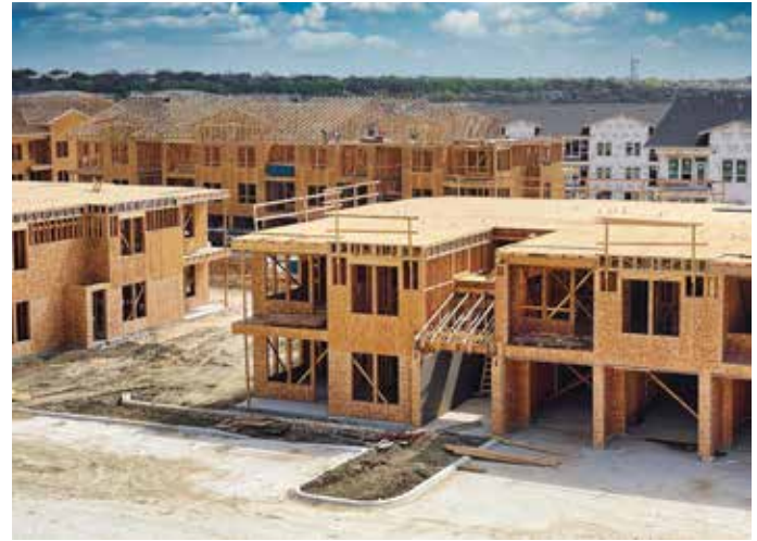
wood sheathing for roof in new construction
