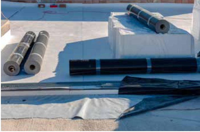
TPO roof – A commonly used flat roof system
