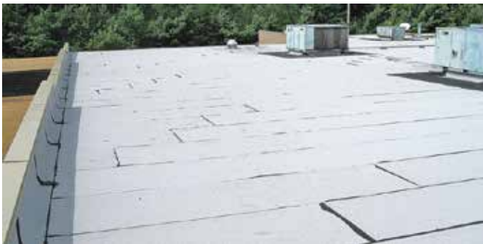
Modified Bitumen roof system – A commonly used flat roof system
