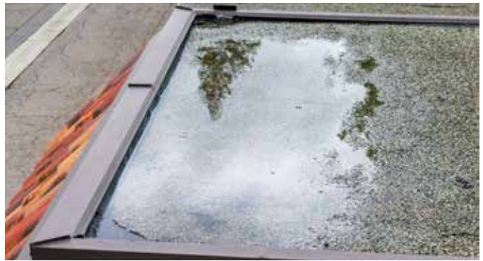
Example of ponding water on a roof
