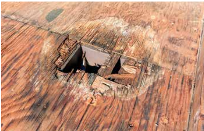
Example of a damaged wood deck that must be repaired
